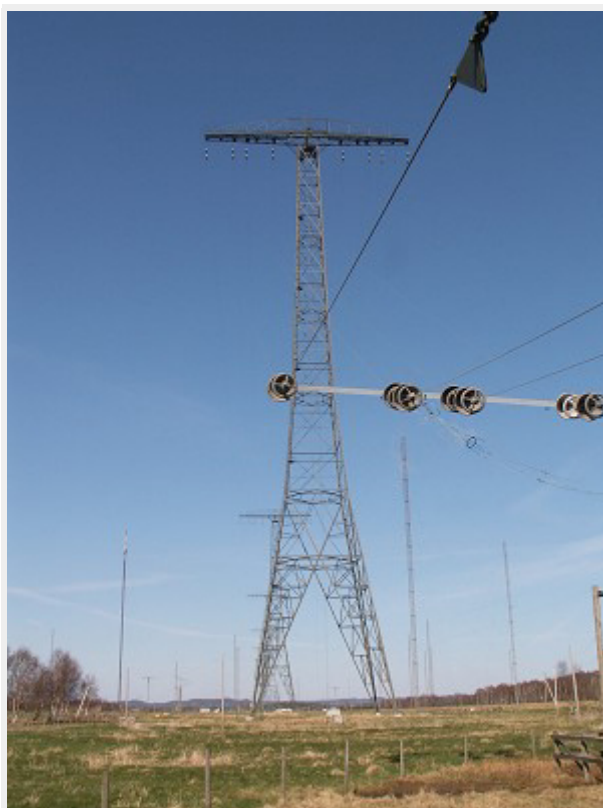
The location of the radio station was carefully chosen to get the best communication across the ocean. The level terrain in the villages Grimeton and Hunnestad outside of Varberg on the Swedish west coast was finally selected as the best to put the six towers.
