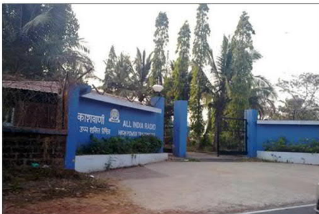
Entrance of SW & MW Transmitter Site
