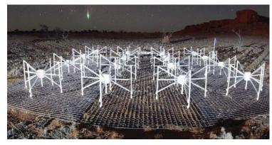
The Murchison Widefield Array (MWA) is a low-frequency radio telescope in Western Australia. The front-end of the MWA consists of 4,096 spider-like antennas arranged in 256 regular grids called 'tiles', spread over several kilometres within the Murchison Radio-astronomy Observatory (MRO).
