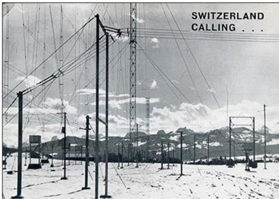
A QSL card from the collection of Bengt Ericson showing the antenna system at the Swiss Shortwave Service received in 1957. The transmitter had the call HER 5 and operated on 11865 kHz.
