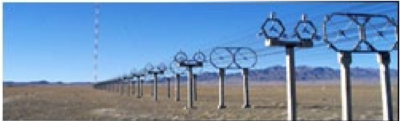
Figure 19: Open feeder line from transmitter to antenna at Dalandsadgab
