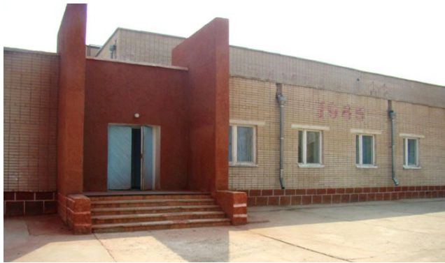
Figure 20: Transmitter housing, Choibalsan
