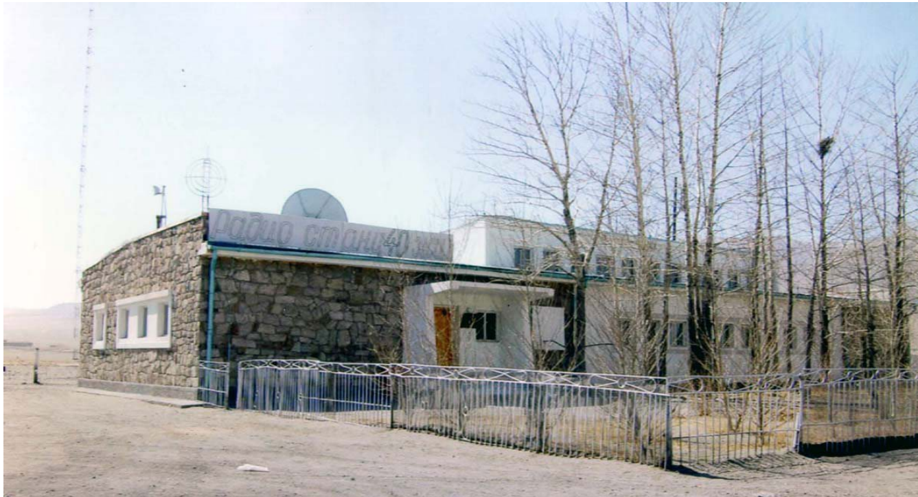
Figure 22: Old transmitter housing, Ölgii
